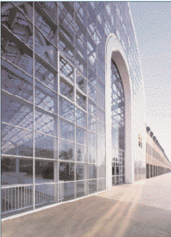
Hall 8, IMEX's new home at Messe Frankfurt
